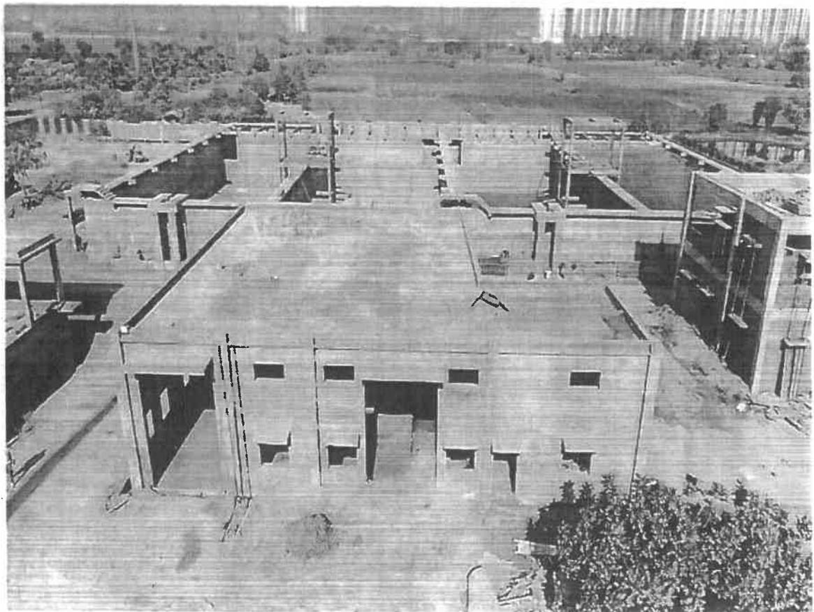
Const of 21.5 MLD STP of Siddhartha vilay 42B
